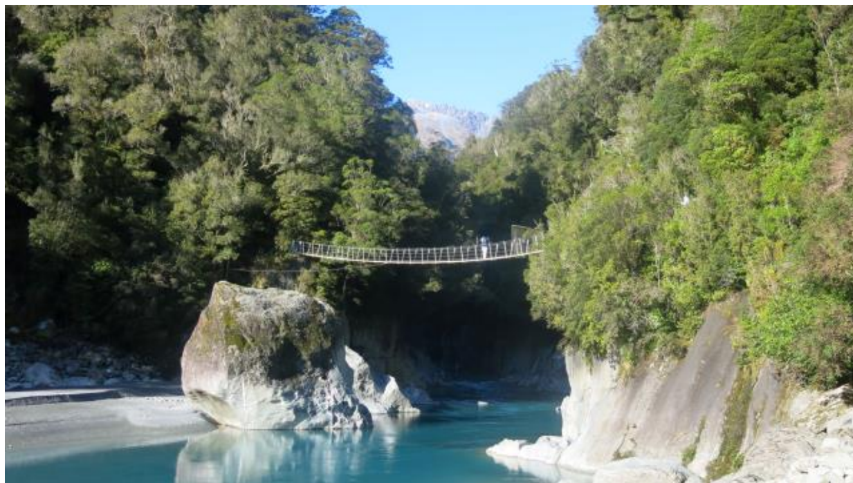
Whataroa River Bridge, photo by Raymond Ford
