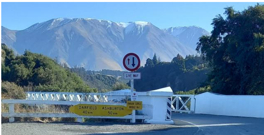
Rakaia Gorge Bridge. Our starting point
