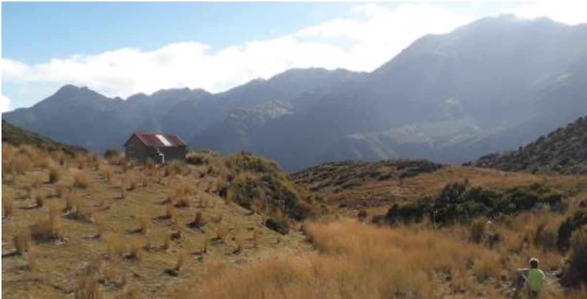
Friday 10:15am. A refurbished Yeats Ridge Hut
