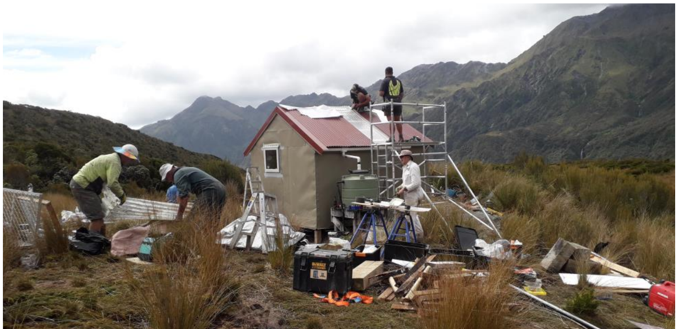
The new roof. Thursday 3pm
