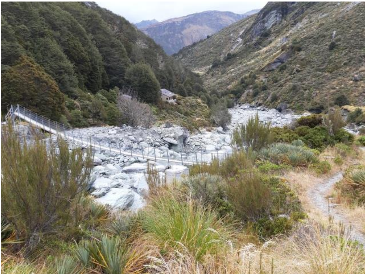
Dart Hut and the bridge over Snowy Creek
